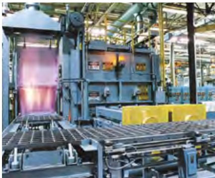
Charge end of a two row pusher skid tray furnace, which is used for high production of similar parts.
